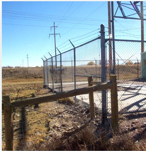
Fencing should never be adjoined to the substation; it can become energized.
