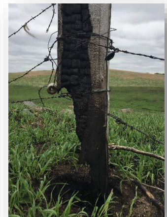
A member reported this burnt pole due to a crop fire.
