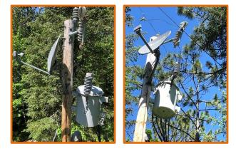
**True Story #2** – The crew found this dish that was installed within 11 inches of the 14.4 KV energized cut out. Crew removed dish and talked to the home owner about the dangers of having it installed on the pole. No items should be attached the pole by a member of the public; it can be dangerous space when you are not wearing proper personal protective equipment and have no experience in line work.
