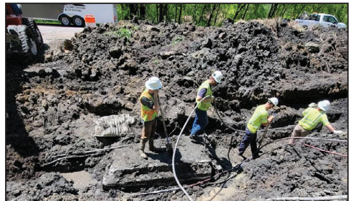
Underground crews work to move and install electric cable for the Highway 14 expansion project in service territory outside of New Ulm. (E)
