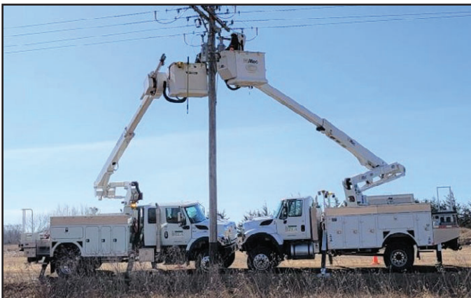
BCREA line crews use two bucket trucks to perform annual maintenance on an Oil Circuit Reclosure (OCR) on a pole.
