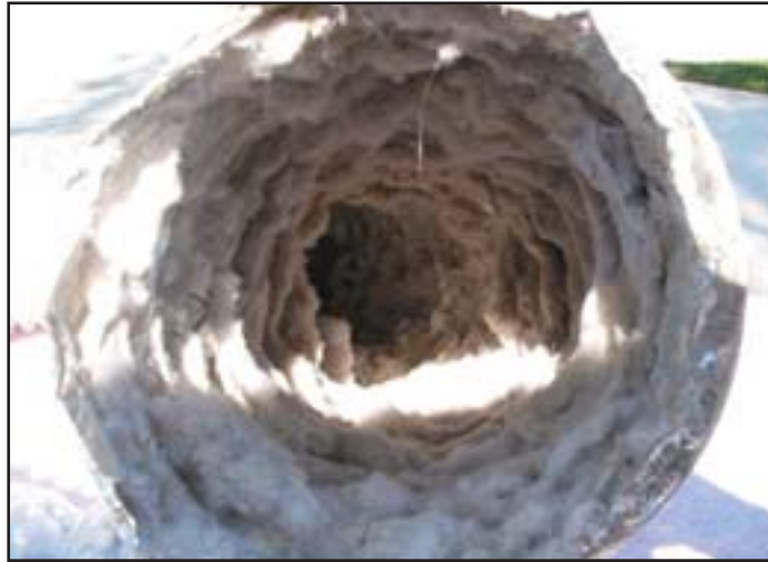
This isn't a cave. This is what the inside of your dryer vent hose may look like if you haven't cleaned it for awhile. This kind of blockage can make your clothes dryer operate inefficiently.
