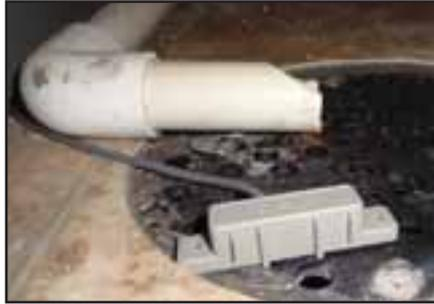
**A flood sensor from Heartland Security gives you the ability to receive a phone call if your sump pump fails and your basement is flooding.**
