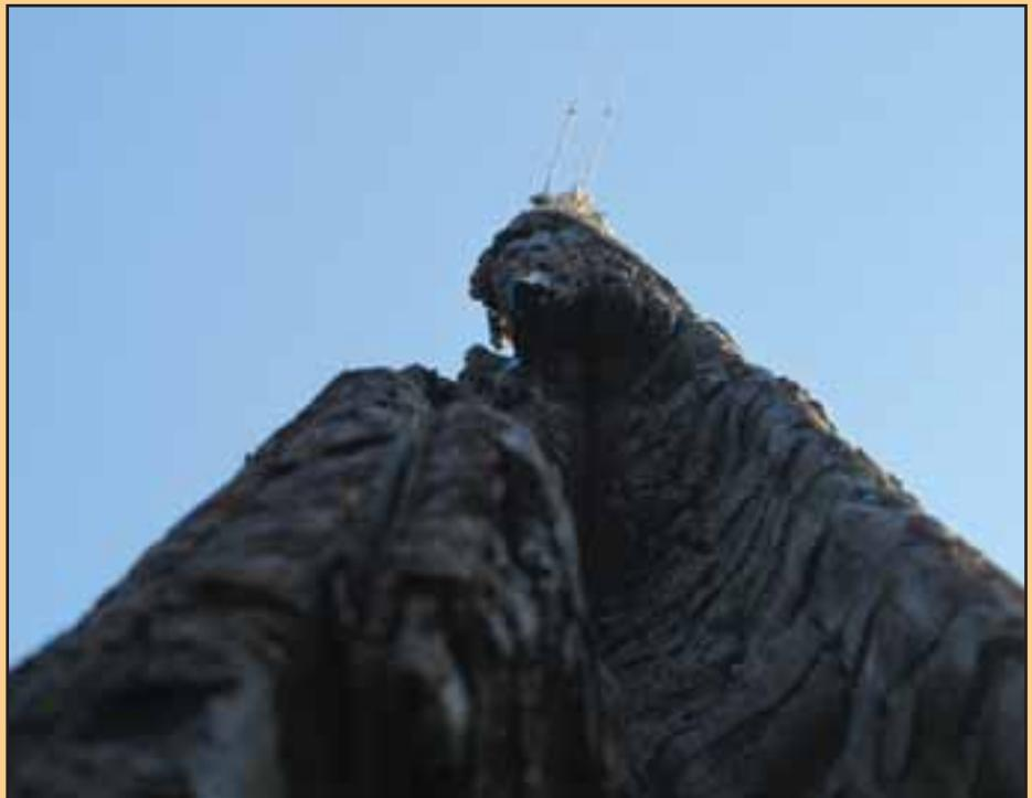
What do these 2 photos show? Nope, it's not a work of art, but the same electric pole that was a victim of a ditch burning. Burn ditches with caution this fall; protect the poles to prevent outages. You will be billed for the cost of replacing a pole and the line crew's labor; this one cost about \$800. (E)
